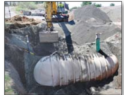
Removal of old underground tanks
